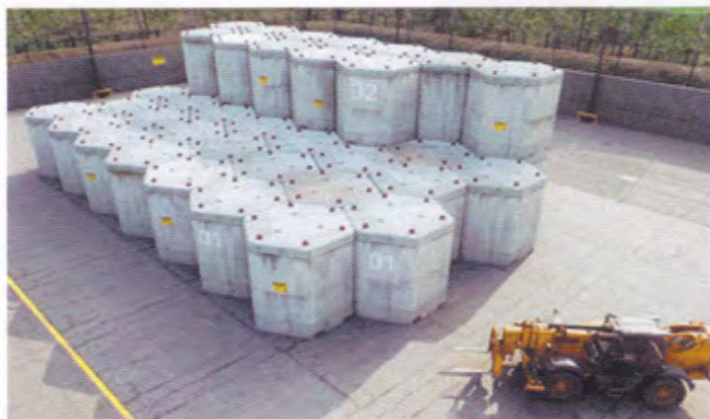
ILW Management – Proposed ILW Storage Array
