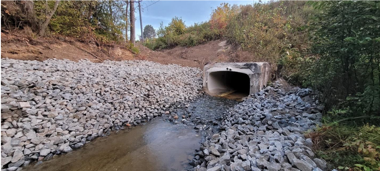
C197 (Etmanskie Swamp Culvert) Rehabilitation
