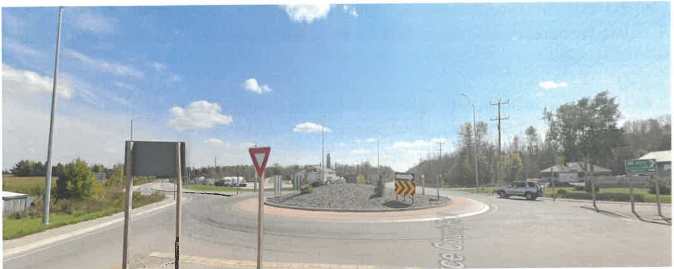
Completed Roundabout Highway 21 and Bruce County Road 10
