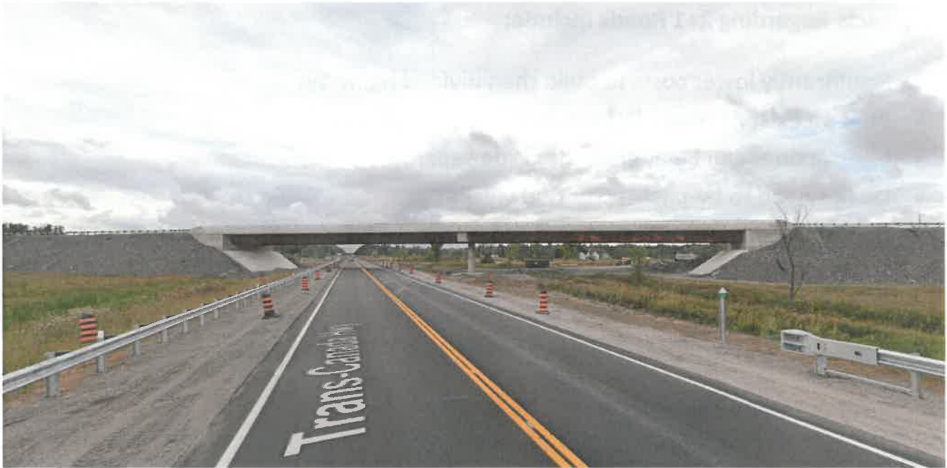
Completed County Road 508 Highway 17 Overpass with Provisions for future four-laning
