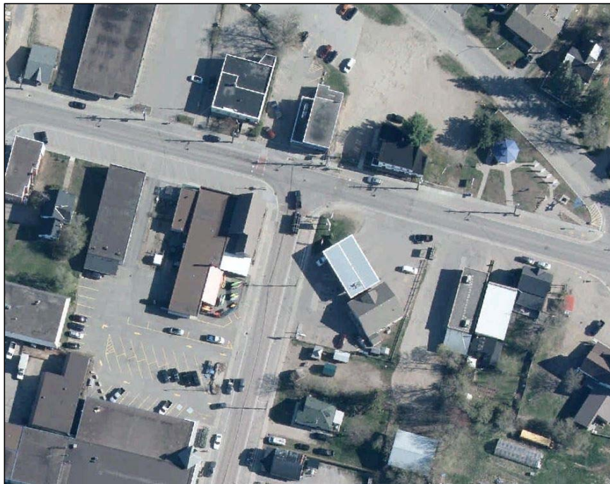
Figure 1-1 Aerial Image of Barry's Bay Intersection
