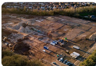
Brownfield Rehabilitation/ Development
