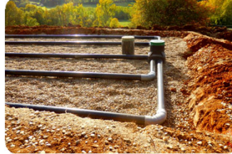
Septic system improvement
